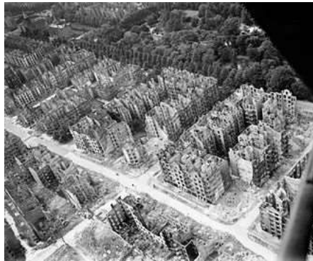
Typical bomb damage in the Eibek district of Hamburg, 1944 or 1945
